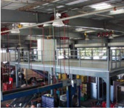
This automotive service center installed our storage platform over their work area to reduce clutter on the ground.
