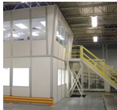
The walls on the top floor of this control room are angled out to provide plant personnel with a better view of the production line below.
