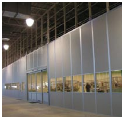
Extra tall walls separate specialized manufacturing equipment into an environmentally controlled area to improve quality control.
