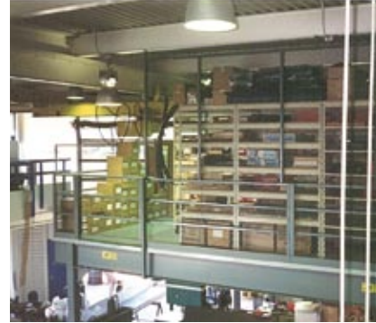
This new storage platform enabled maintenance staff to expand their existing storage area without losing valuable floor space below.
