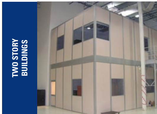
This two story modular building was constructed without the mess and disruption commonly associated with conventional construction.
