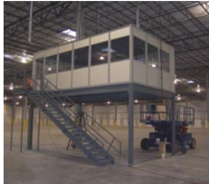
This plant manager's office was built on top of this mezzanine to aid in supervision of plant personnel and equipment.
