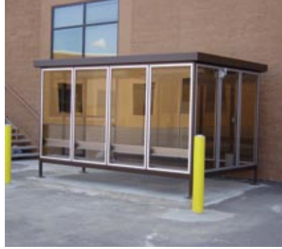
12'x9' Smoking shelter with an aluminum bench and photocell activated interior lighting.
