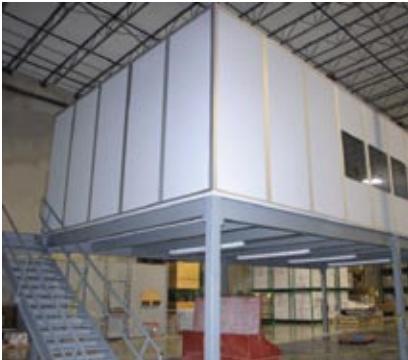
This elevated modular office was installed on this mezzanine to create a training facility that enables trainees to learn by easily observing plant operations below.
