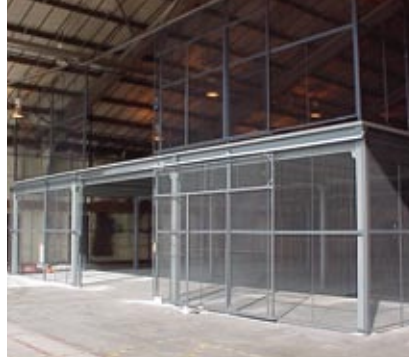
Secured storage space is created above and below the mezzanine deck surface in this Air Force Base hangar.
