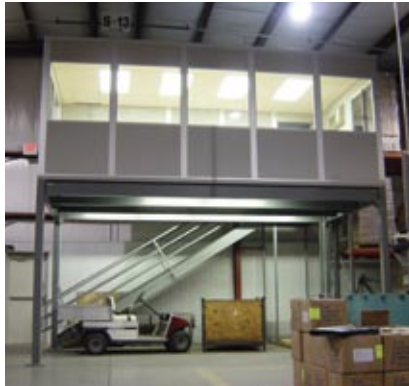
This modular system was integrated with our mezzanine to create a new office space while keeping the floor below open.
