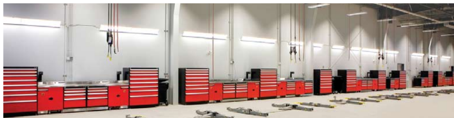
Capital Pontiac - Service Equipment (SK)
